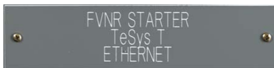
Standard Unit Nameplate
