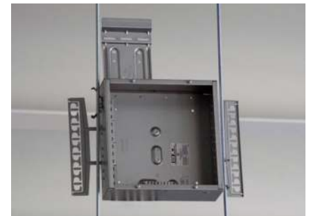
Grand Slam Box installed using Multi Function Clips
