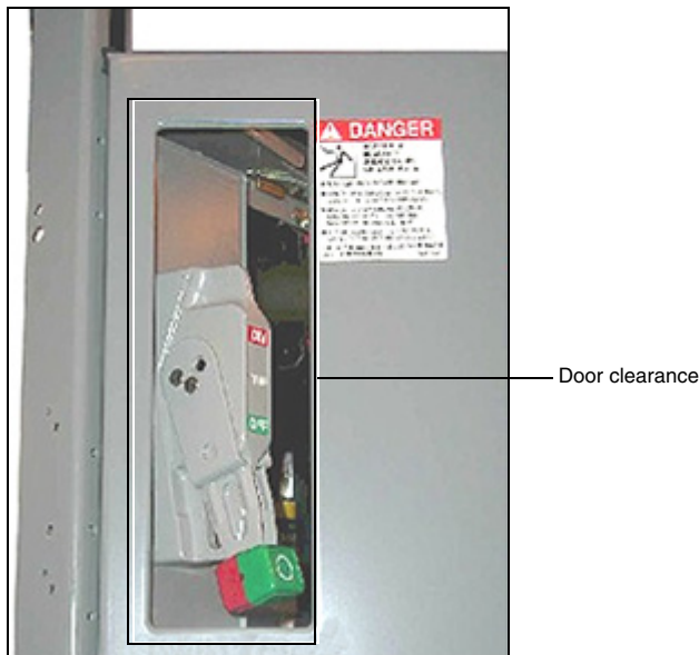
Figure 3: Handle–Operator Door Clearance
