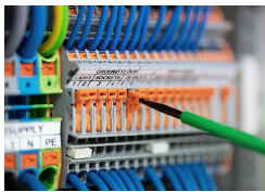
Pivoting a knife disconnect.
